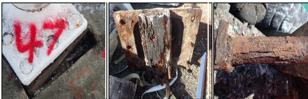
Figure 11 Decaying timber and corroded bolts supporting bollards 47 (left) and 46 (centre and right)
