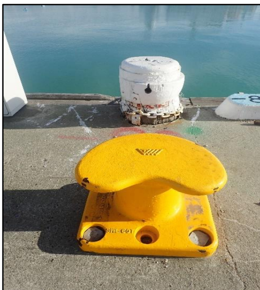
Figure 13 Newly installed steel bollard
