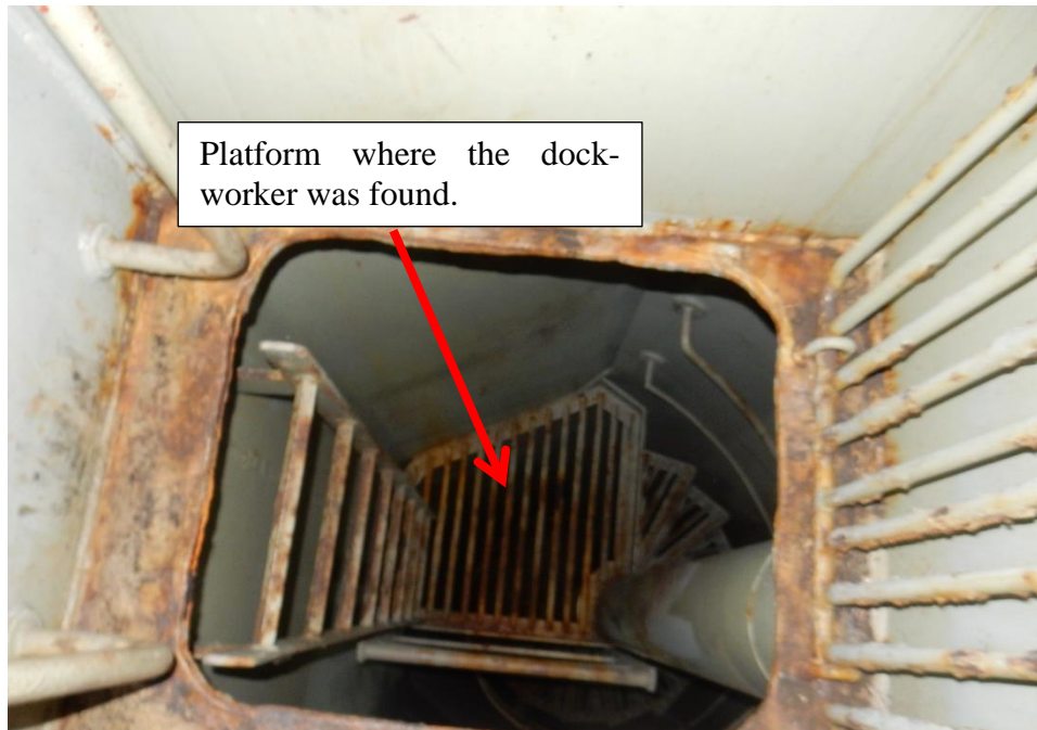
Figure 4. Entry hatch to cargo hold 7.
