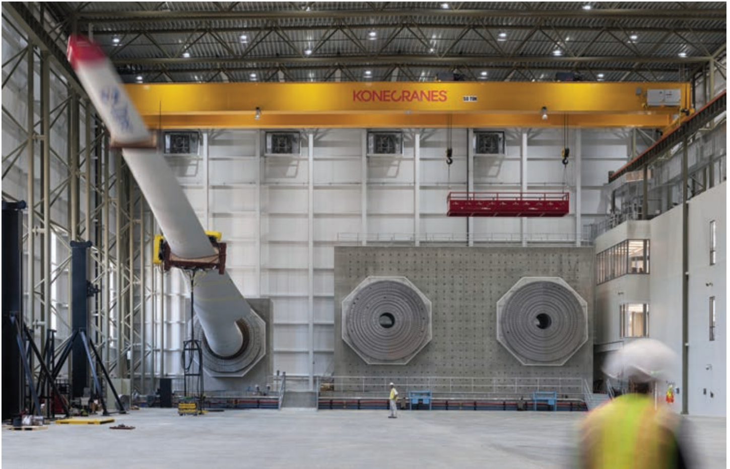
Figure 8. MassCEC's Wind Technology Testing Center (WTTTC). (image credit: Chuck Choi 2011)
