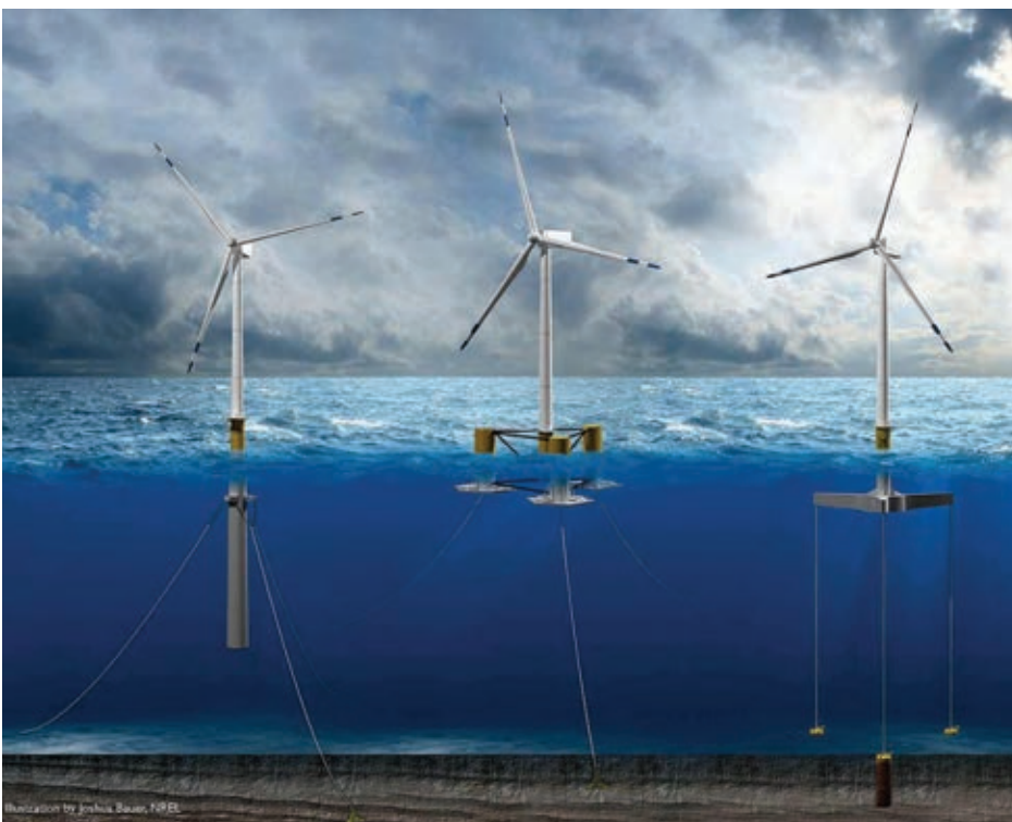
Figure 14. Floating concepts push technology development farther offshore. (image credit: Josh Bauer, NREL).
