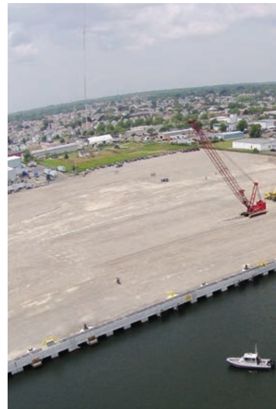
Figure 16. The New Bedford Marine Terminal is a facility that supports Jones Act 1 compliant logistics by supporting the world's largest land-based cranes at the quayside. (photo credit: MassCEC)
