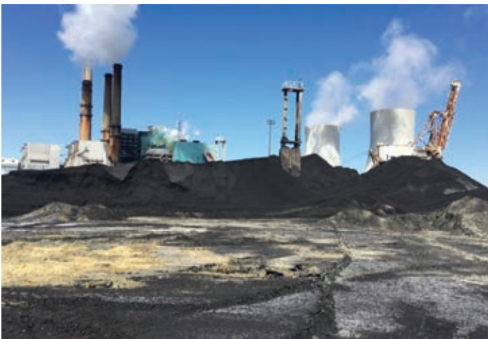
Figure 5. Brayton Point, New England's largest coal-fired electricity generation plant retired on June 1, 2017. Shown here are the last remnants of the facility's 680,000 ton coal pile in March 2017.
