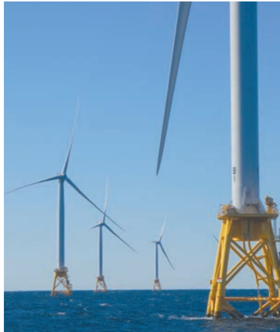
Figure 4. The 30 MW Block Island offshore wind demonstration project, developed by Deepwater Wind. (Image Credit: MassCEC)
