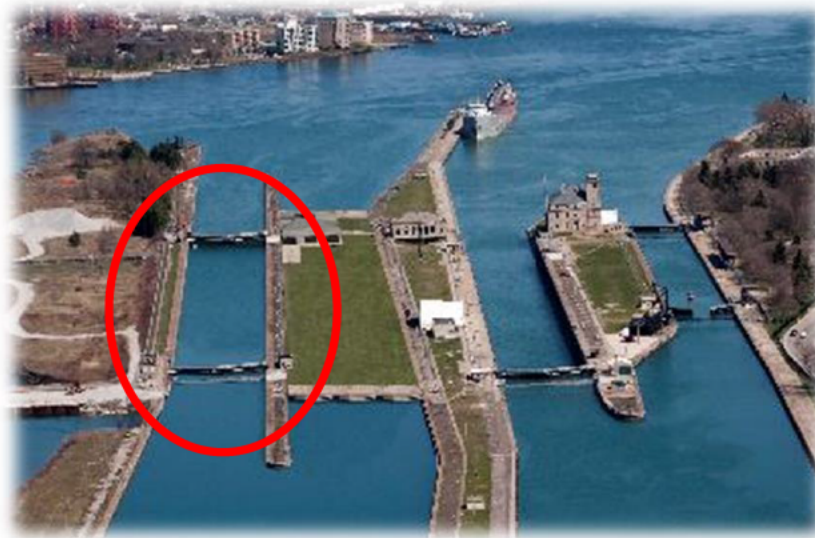
Figure 12. Conceptual rendition of the Proposed “Poe-sized” lock in the Davis and Sabin Lock Footprint
