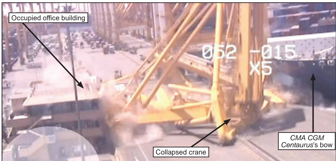
Figure 9: Crane collapsing in close proximity to an occupied office building
