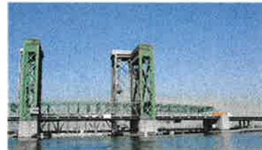
The Henry Ford Bridge runs parallel to the Heim Bridge and carries trains across the Cerritos Channel to Terminal Island and the ports of Los Angeles and Long Beach.
