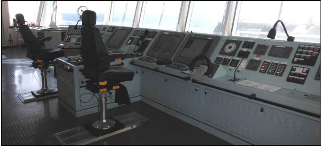
Figure 2: Wheelhouse and layout of navigation equipment
