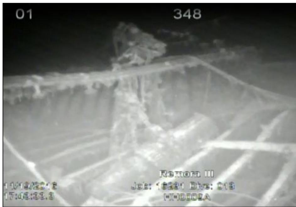
Figure 44 Collapsed iron windlass with chain connected to iron capstan on forecastle deck (ATSB)
