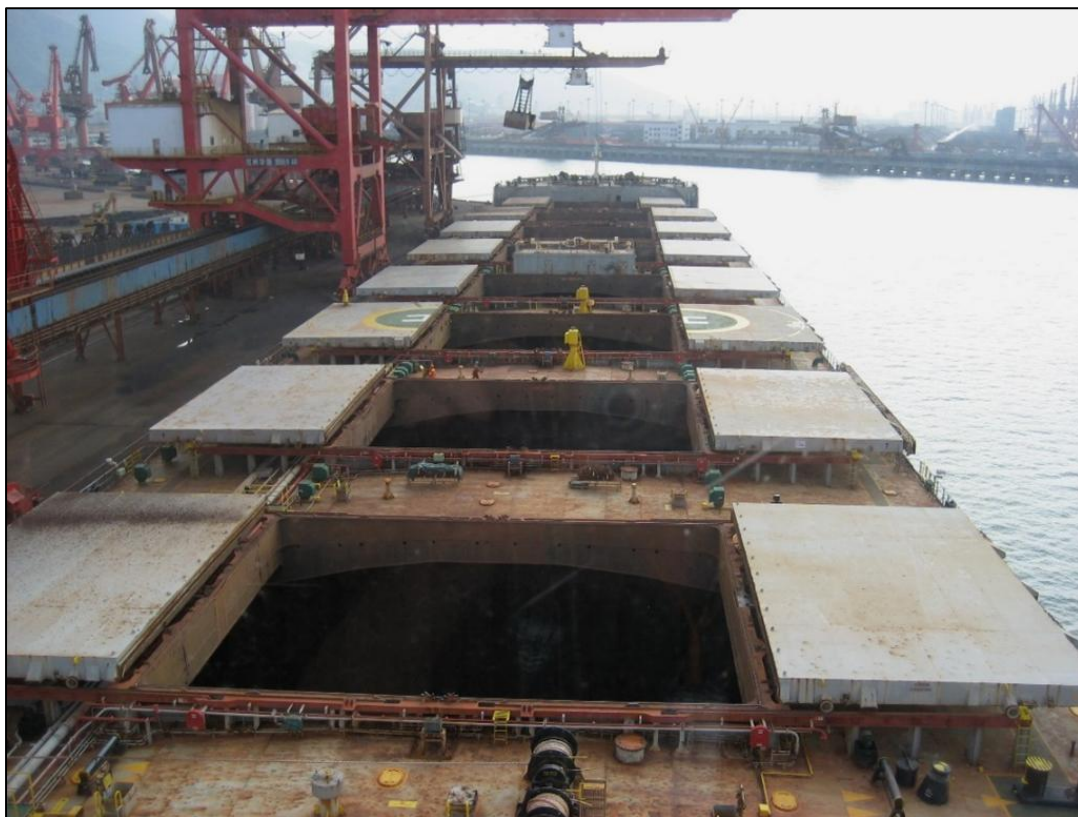
Figure 1: General view of Abyo Audrey from the bridge
