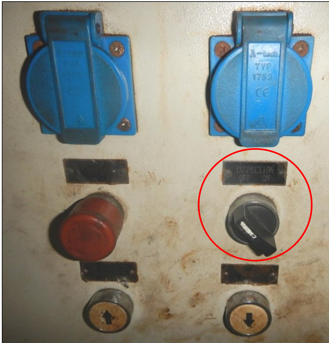
Figure 7: Inspection switch (in the OFF position)
