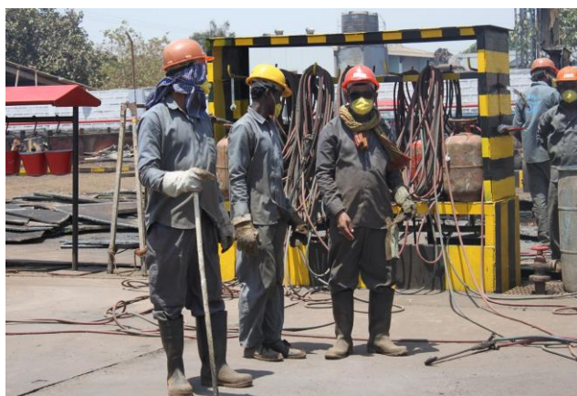
JRD yard_HKC ClassNK certification in progress (©ECSA - 29.04.2016)
